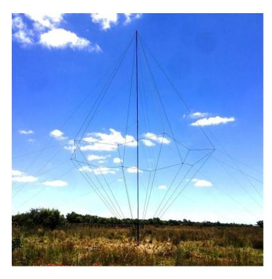
The BCM330 is a wideband, high power HF conical monopole antenna that exhibits an omni-directional, high gain radiation pattern.
